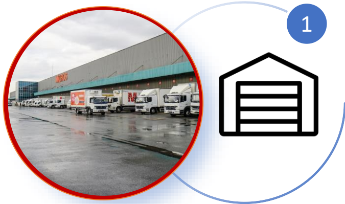
Distribution Centers expansion
